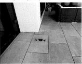
June 25, 2021, Photo Disc 1, Photo 9; the IRC requires impervious surfaces within 10-feet of the building foundation to slope a minimum of 2-percent away from the building. This slope was consistently measured to be less than this required minimum.
